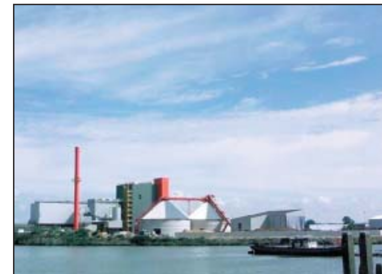
Co-generation plant (Siemens AG)
