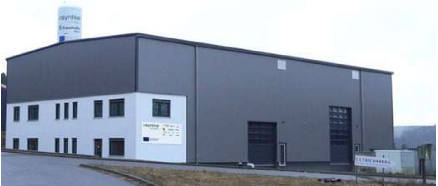
Pilot plant for the To-Syn-Fuel project in Markt Hohenburg, district of Amberg-Weizsäcker. Credit: Fraunhofer UMSICHT
