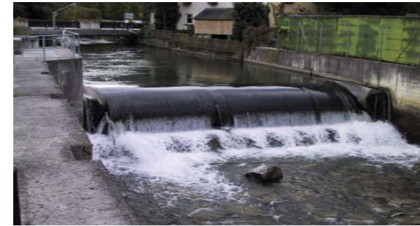
Small hydro power installation. Source: ESHA
