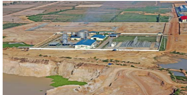
CHP installation. Source: COGEN Europe
