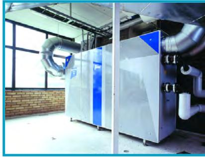
Fig.5: Turbec T100 installed in a boiler room (by courtesy of Turbec)
